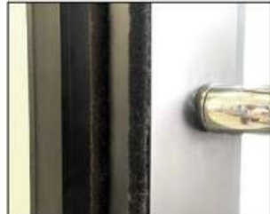
Door Pile Weatherstrip Applied on Door Astragal.
